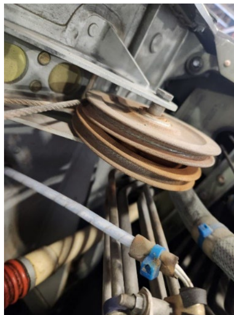
Figure 1 – installation de poulies
